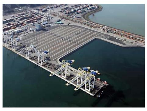
DP3 has increased the capacity at Deltaport by up to 600,000 TEUs (twenty-foot equivalent units) by adding a third berth and 20 hectares of container storage facilities to the existing two-berth container terminal.
