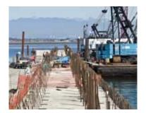
Construction workers install the caissons, the large cement dock structures, which create the foundation for the third berth. Port Metro Vancouver to accommodate consumer and business-driven
